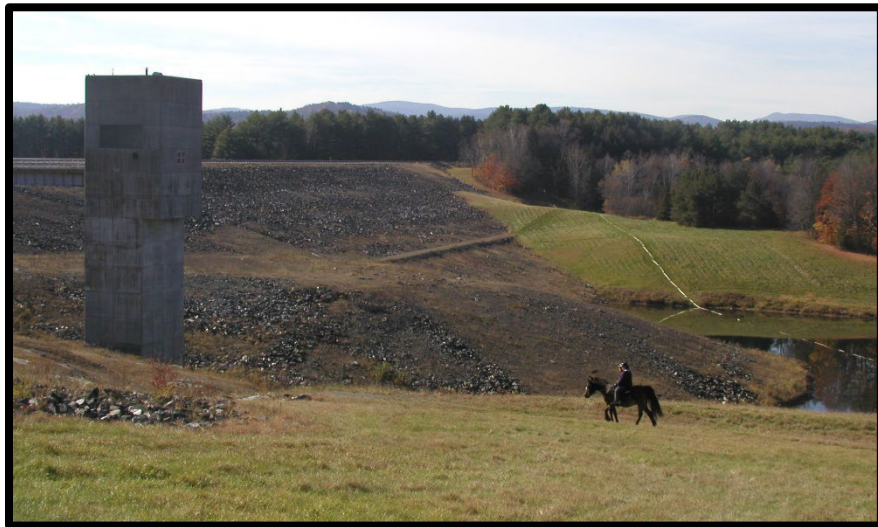
Photo 5.2 Side View of the Dam
