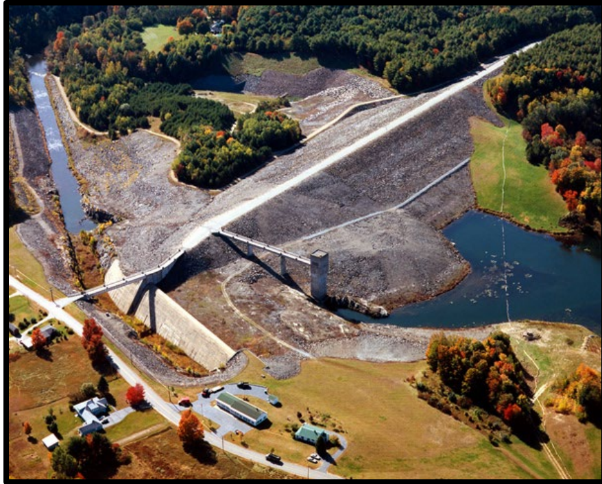
Photo 5.1 North Springfield Dam Access
